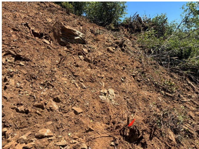
Figure 4: Terrain at point of rollover
